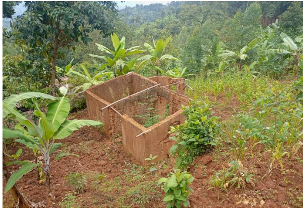
3.6.A. Abandonment of homes due to landslides
